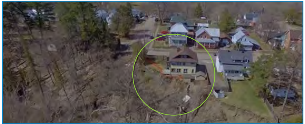
CLUOV's Moffat Street property had issues with erosion this spring.
